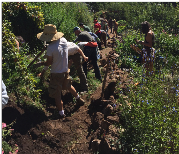
Clearing the way for rebuilding one of the Garden’s rock walls.
